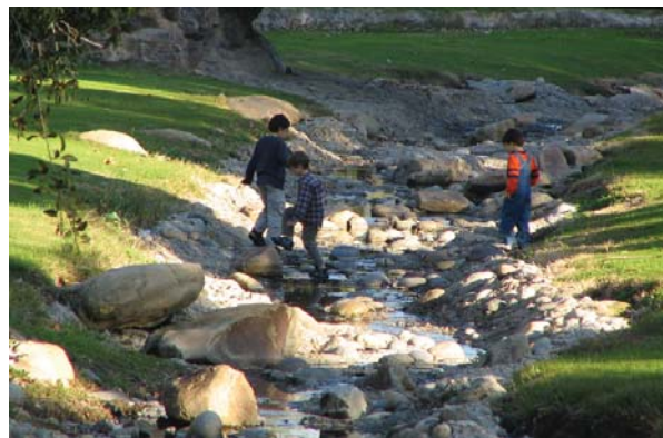
AN EXAMPLE OF A CONSTRUCTED CREEK DIVERSION
